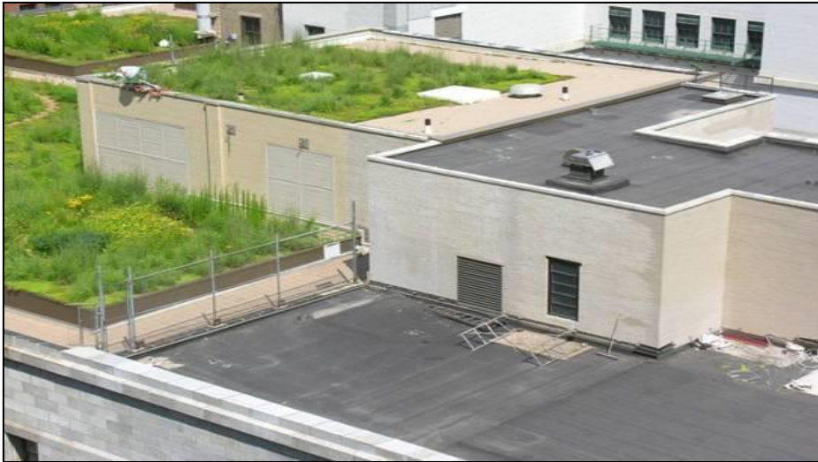
Chicago City Hall green roof and adjacent building with black asphalt roof.
