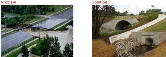
A 2005 storm in Toronto caused \$647 million in damages including destruction of this culvert (left), which was replaced with a larger, more resilient culvert (right). Source: Toronto Environment Office).
